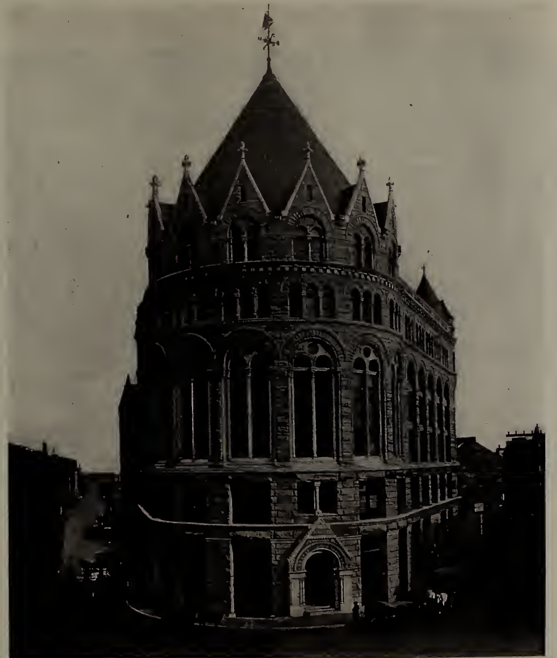
BOSTON CHAMBER OF COMMERCE, India Street and Central Wharf. Erected 1890-92, at a cost of $400,000, from plans by Shepley, Rutan, & Coolidge, successors to Richardson.
